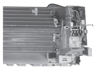
Remove 1 screw from control board complete. Then pull out the control board complete.
